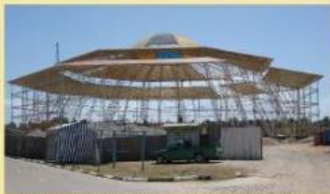
J.C.C GLASS SANCTUARY DURING CONSTRUCTION
